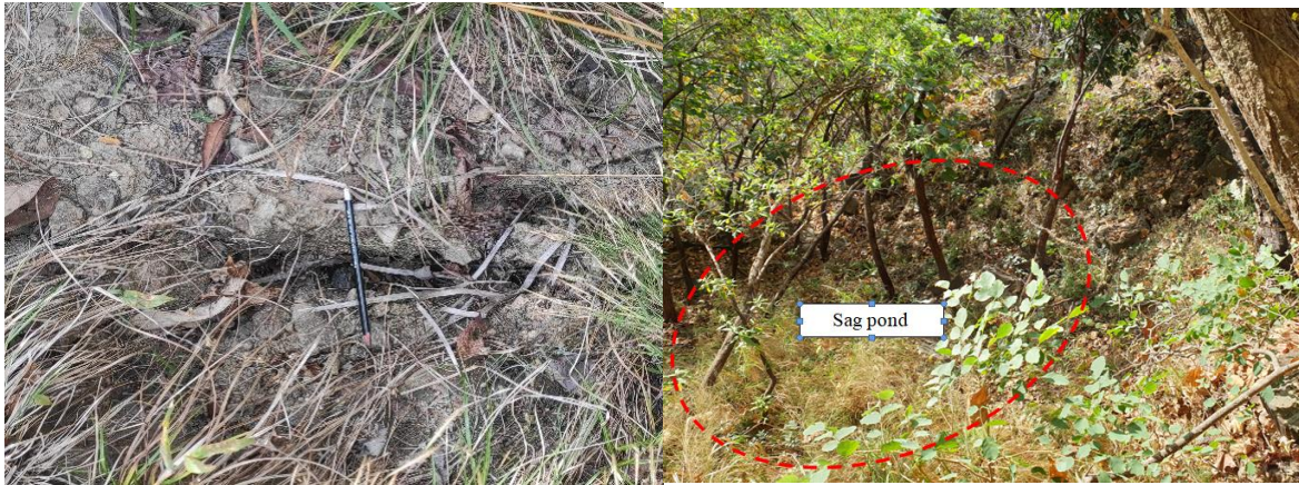
Figure 2 Cracks parallel to movement and present sag pond at the top portion
