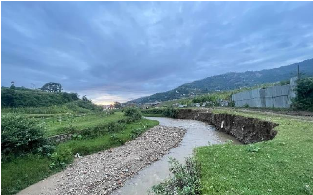
Photograph 1: Erosion and deposition by Triveni River at Dahachowk.
