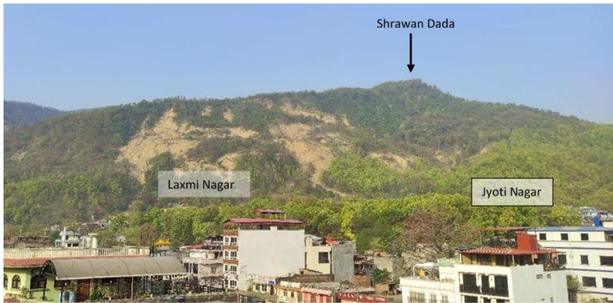
Figure 1 Photograph of Jyotinagar Landslide from Butwal city
