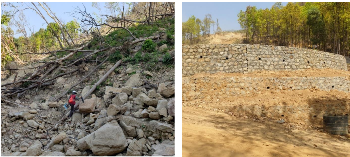
Figure 3 Drunken trees and gabion wall inside the landslide mass
