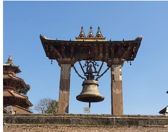
Figure 10: Metal bell hung in between two big carved sandstone pillars at Patan Durbar Square
